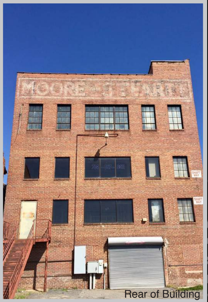
Front of Building
